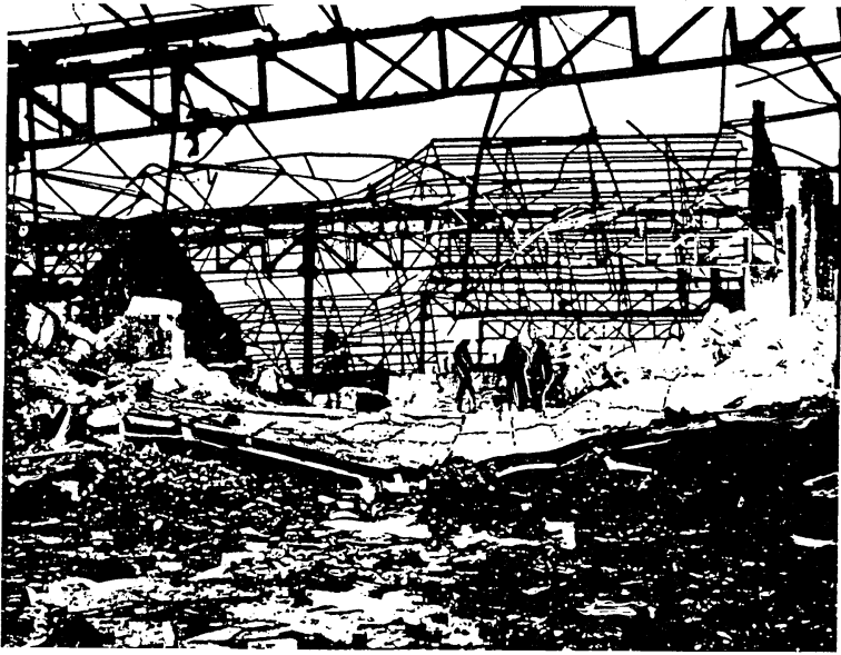
Figure 2 The warehouse after the explosion
