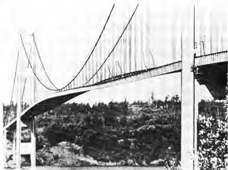
Figure 16 Wind-excited asymmetric torsional oscillations of the first Tacoma Narrows Bridge. Bulletin 116, University of Washington Engineering Experiment Station.
