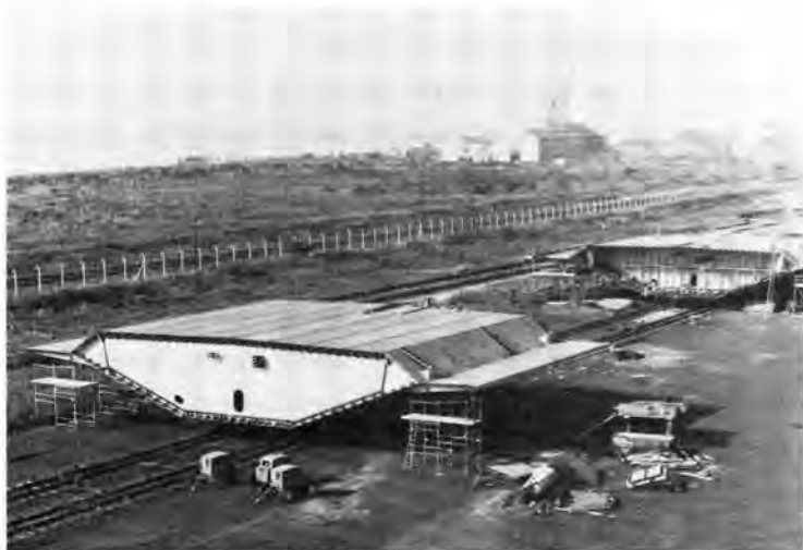
Figure 6 Construction of a box section. Donald Innes.
