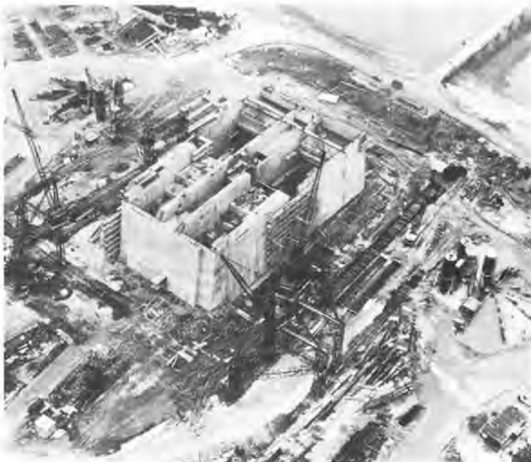
Figure 5 Barton anchorage nearing completion. The upper block is 65 metres long by 37 metres wide by 22 metres high. Including its 36 metres deep foundation structure. The mass of the anchorage is about 300 000 tonnes. Handford Photography.
