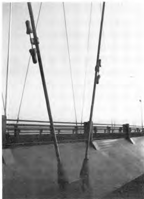
Figure 13 (left) Stockbridge dampers on the Humber Bridge. Colin Price.
