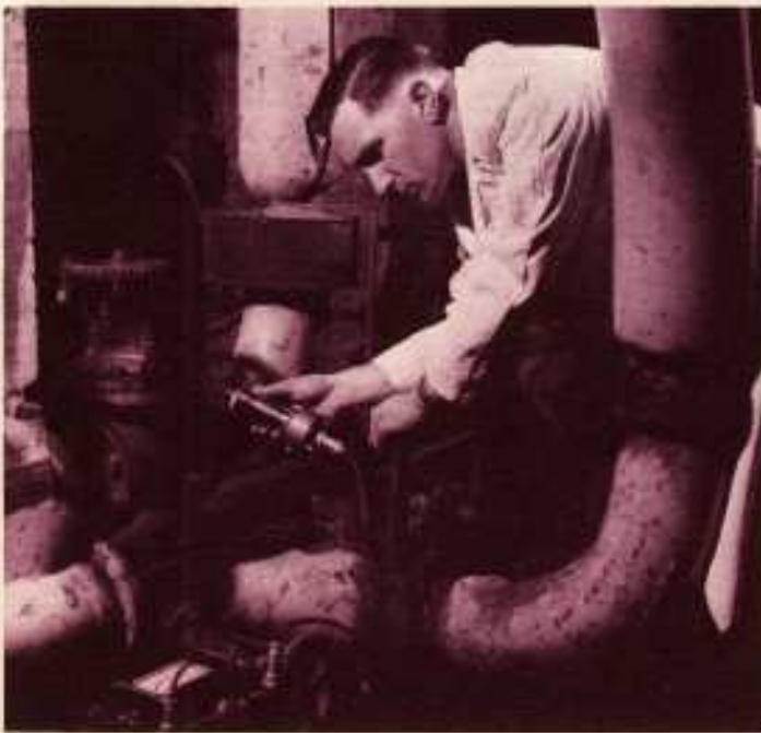
A gauge being used to measure the thickness of a pipe. U.K. Atomic Energy Authority
