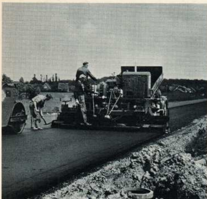
Laying a road with bitumen.
