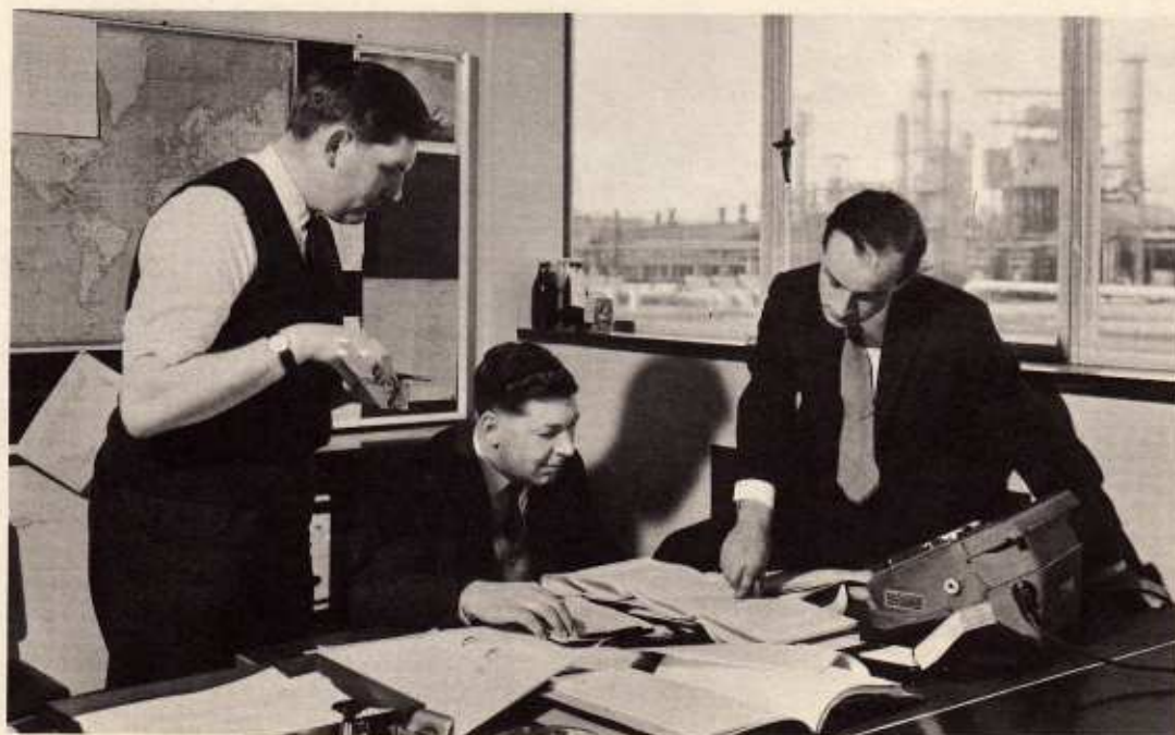
Days of discussion precede the expensive business of building plant to manufacture a new chemical. The need for the new chemical must be established, the quantity in which it will be required, and the best way of manufacturing it.
