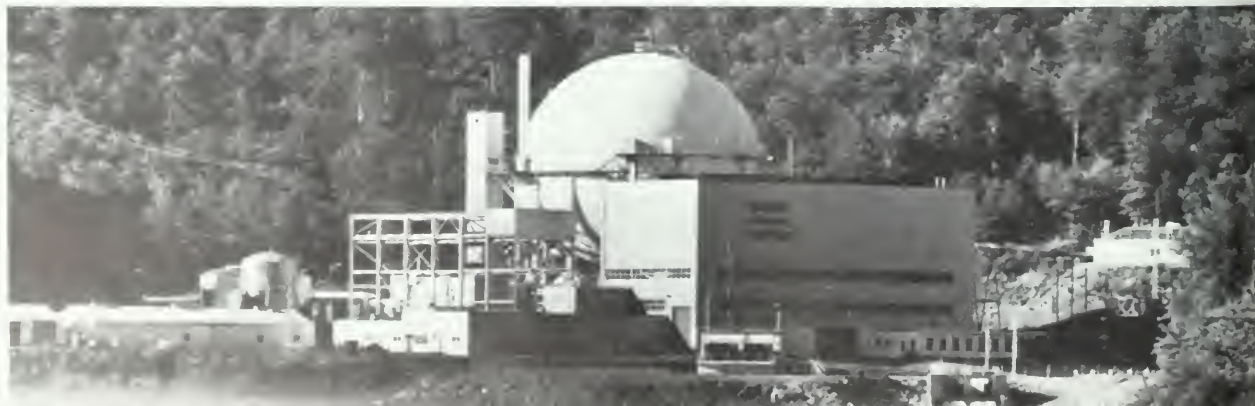
The Yankee Atomic Electric nuclear power station in Rowe, Massachusetts, which has been producing electricity with a capacity of 175,000 kW since 1961.
