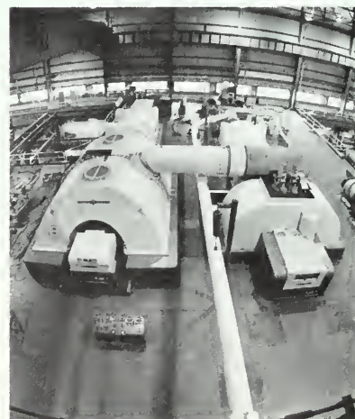
A commercial generator. As in almost all large generators, the coils of wire in which current is induced are around the outside, and electromagnets are rotated on the inside.
