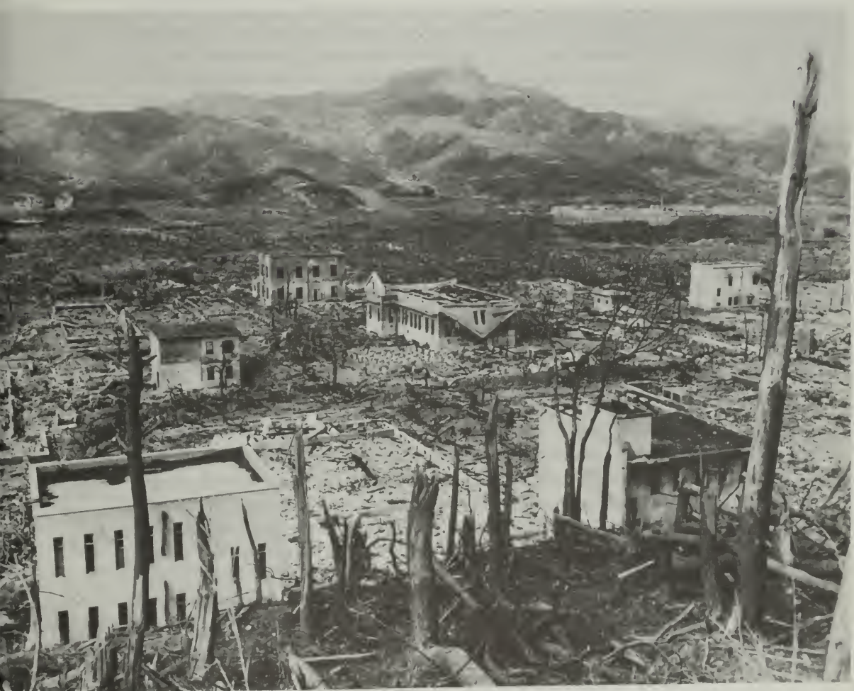
Fig. 18.1 Remains of the Nagasaki Medical College after the A-bomb drop on August 9, 1945. (Photo courtesy of the United States Atomic Energy Commission.)
