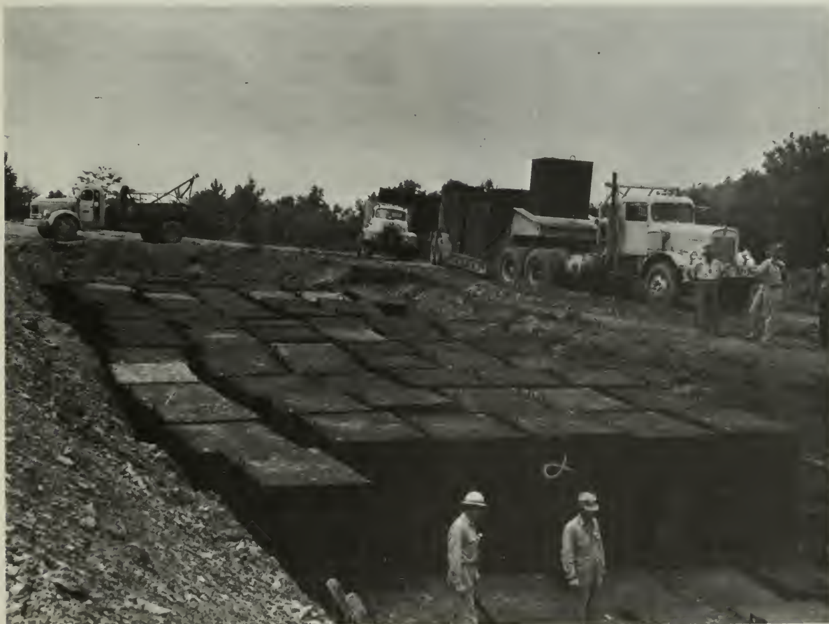
Safe disposal of radioactive wastes with long half-lives is becoming a significant problem. Here steel cases containing dangerously large amounts of radioactive wastes from nuclear reactors are being buried.
