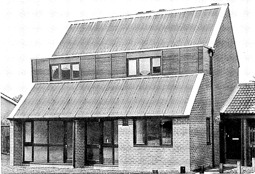
A solar house in Milton Keynes, Buckinghamshire. The solar panels cover the especially large surface area of the roof. The house is also very well insulated.
