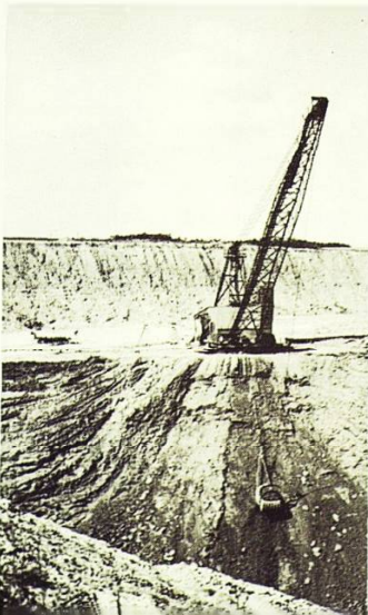
Left: Clay scooped out with a drag line and bucket Centre: Brick presses, each cutting two bricks at a time Right: A large brick kiln being filled with bricks
