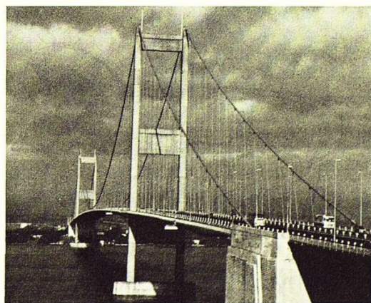
The Severn Bridge is a suspension bridge. It has a span of about 1000 metres.
