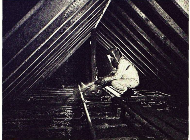
This photo shows mineral fibre being 'blown' into place.
