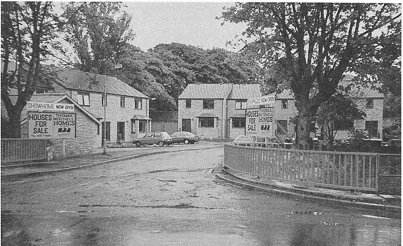
Figure 3 These stone houses are built with a timber frame. The outer walls are made of simulated stone
