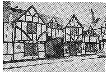
Figure 9 Traditional timber-frame construction
