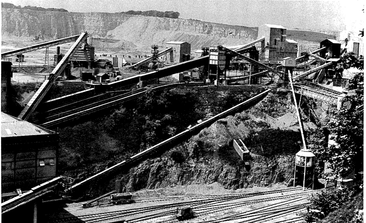
Figure 5 Limestone processing equipment at a large quarry in the Peak District
